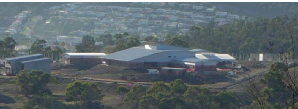
The Wilfred Lopes Centre for Forensic Mental Health nearing completion
