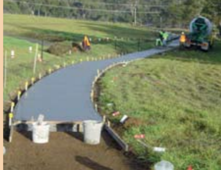
Footpath under construction
