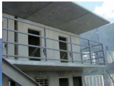
Maximum security cell block under construction
